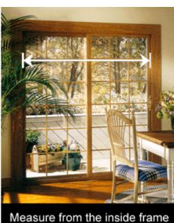
Measure from the inside frame of the door from side to side
